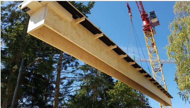
Figure 11: A prefabricated 23,80m roof element on the crane
