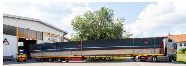
Figure 9: Two roof elements loaded on the truck
