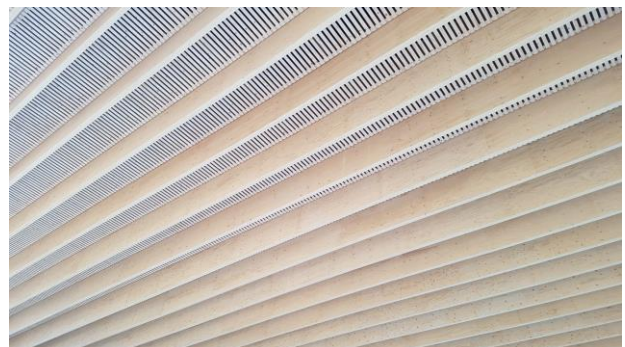
Figure 14: Roof underside with acoustic ceiling and LVL-Panels in visual quality
