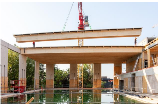
Figure 12: Assembly of the roof with individual LVL \pi -Panels
