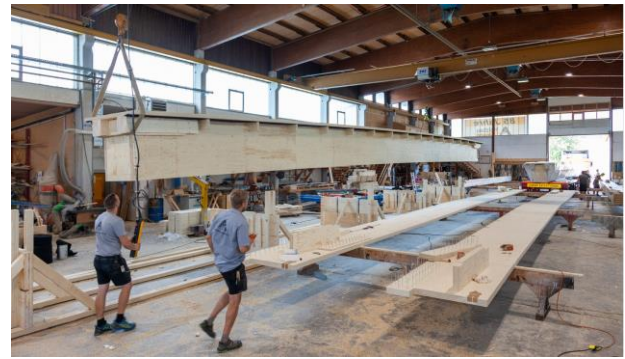
Figure 8: Production of the \pi -elements in the factory
