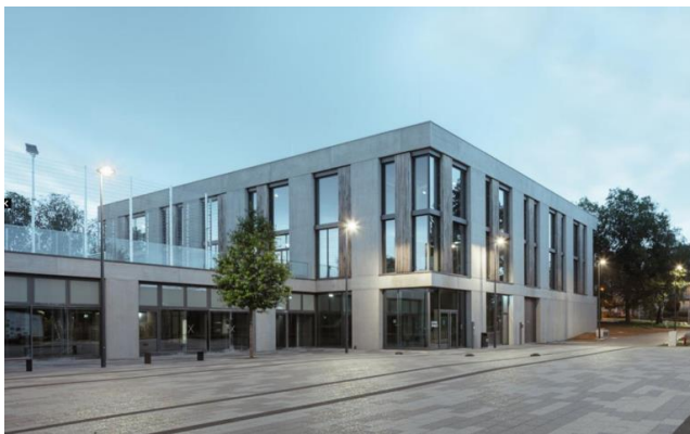
Figure 1: Exterior view of swimming hall within the school campus
